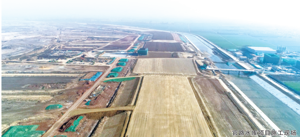
围坝开挖、土堆转运
